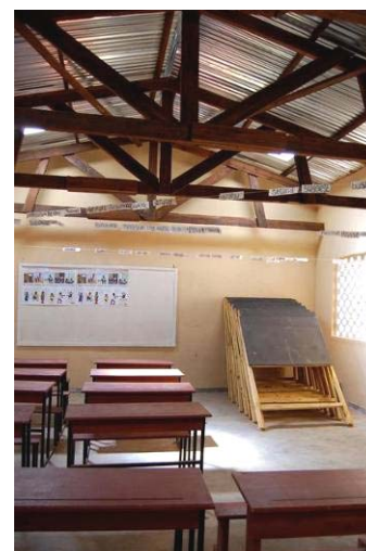
Newly rehabilitated classroom in Mwandama.
