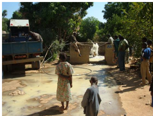
Testing a borehole in Tiby.
