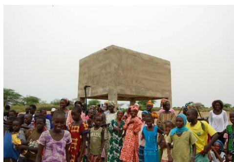
Water tank in Potou.
