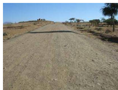
Improved section of the Hawzien-Megab Road in Koraro after rehabilitation (Ethiopia).
