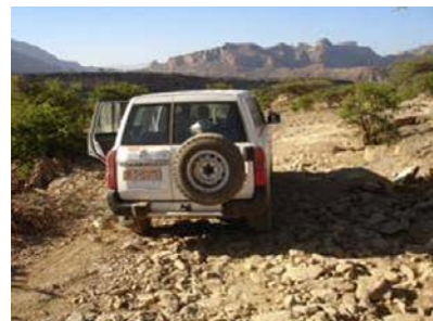
Road conditions in Koraro (Ethiopia) before rehabilitation.
