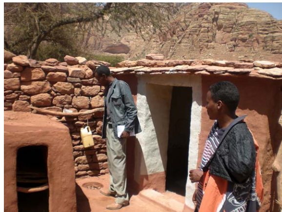
A model house for the sanitation program in Koraro. Pictured here (left to right) are a hen house, hand-washing station, and ventilated improved pit latrine.
