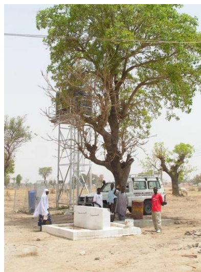
Solar-powered borehole in Pampaida.
