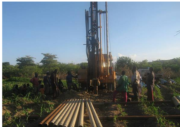
Aqua Well Drilling Co. equipment arrived in Mbola in December 2009 to begin drilling seven boreholes.
