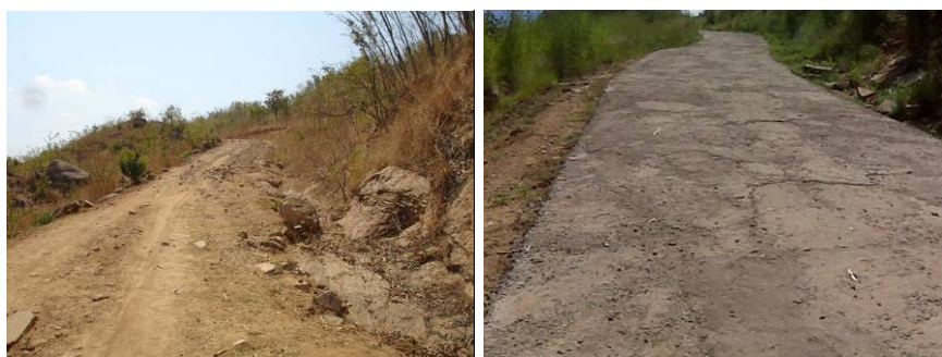
A road in Mwandama (Malawi) before rehabilitation (left) and after.
