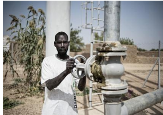
Amadou Coumaré maintains the drinking water supply in the Millennium Village of Tiby (Mali). This solar-powered water pump feeds the MV's piped water system.
